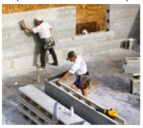
or even a combination of horizontal and vertical assembly is possible. The system of cavities always fits, as the distance between the horizontal cores is equal to the width of the element. The elements are lined up and the wall is stressed together with rebars or
