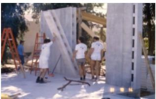
53 dB (12" wall with plaster on both sides); more than sufficient even for separation walls between apartments.
