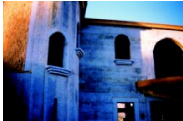
Figure 5.29 RASTRA® used for window trim.
