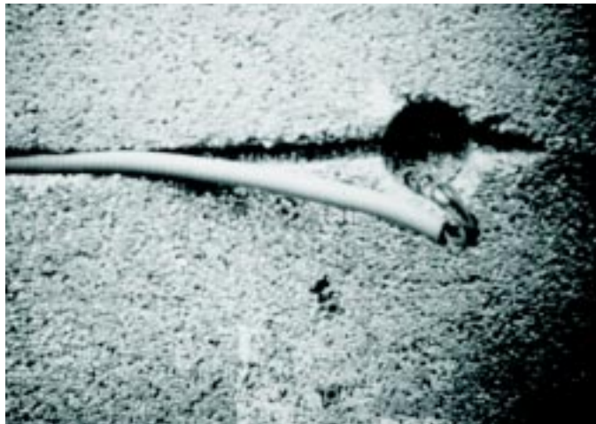
Figure A.4 Closeup of conduit installation in progress.
