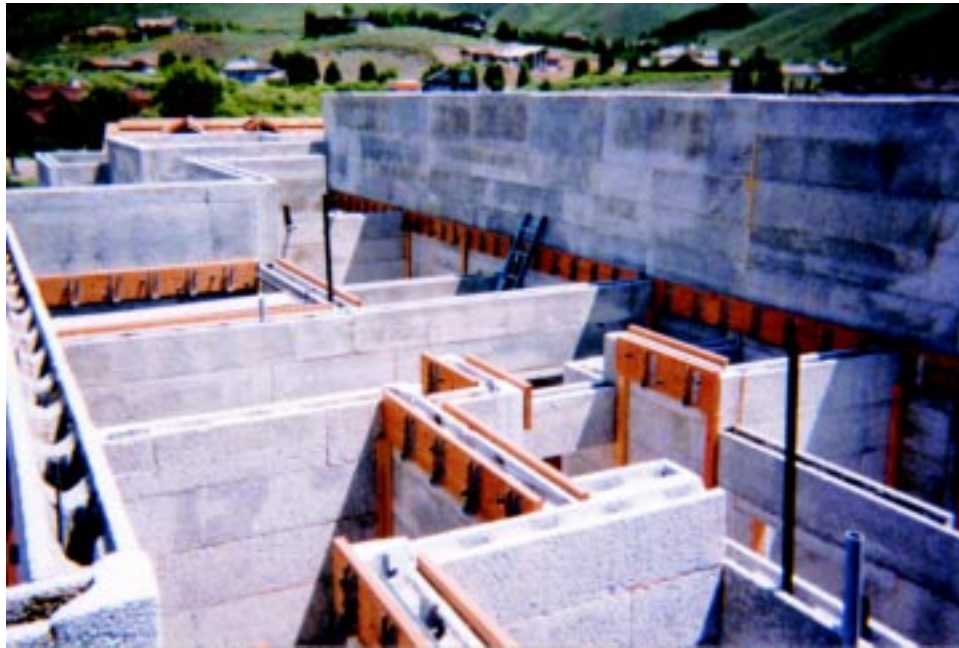
Figure 4.3 Ledgers in place prior to grouting of wall.
