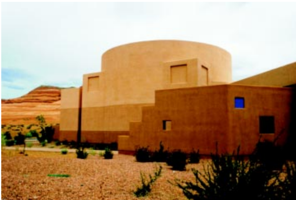
Figure 8.12 Curved wall and architectural elements.
