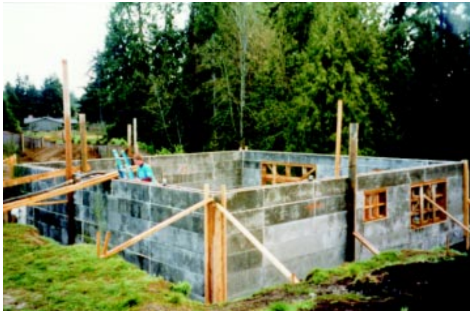
Figure 3.7 Basement wall with bracing prior to grouting.
