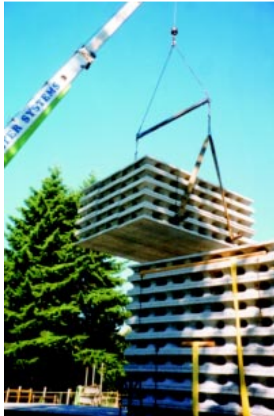
Figure B.3 Unloading RASTRA® elements using a boom crane.
