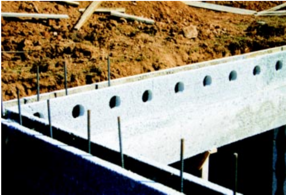
Figure 4.1 RASTRA® wall with cutouts prepared for ledger/anchor bolt installation.
