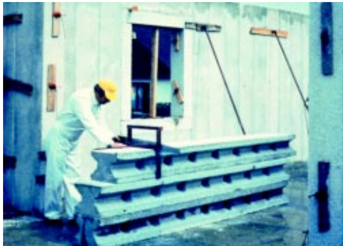
Figure 2.5 RASTRA® saw guide for cutting elements.
