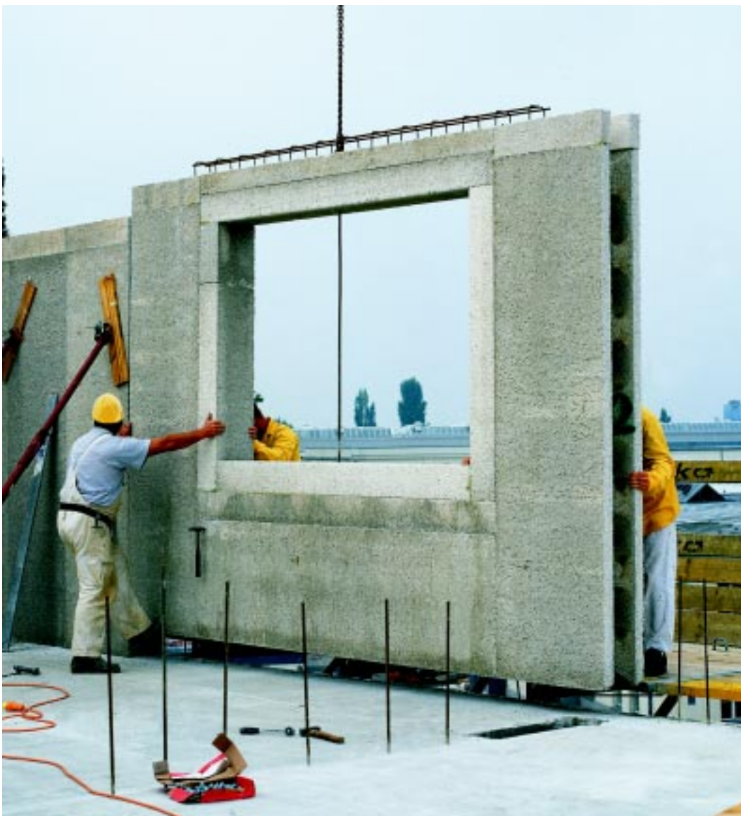
Figure 8.16 Prefabricated panel being lowered into place.
