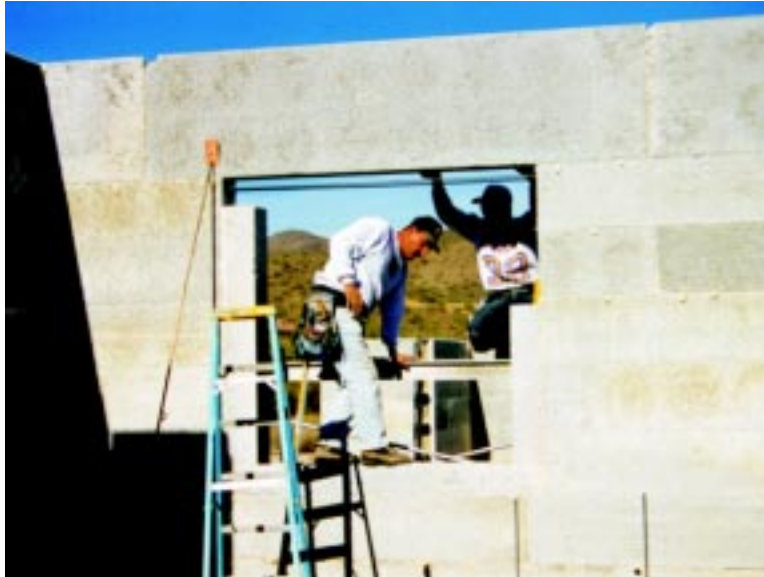
Figure 5.16 Framing window opening with RASTRA® end elements.
