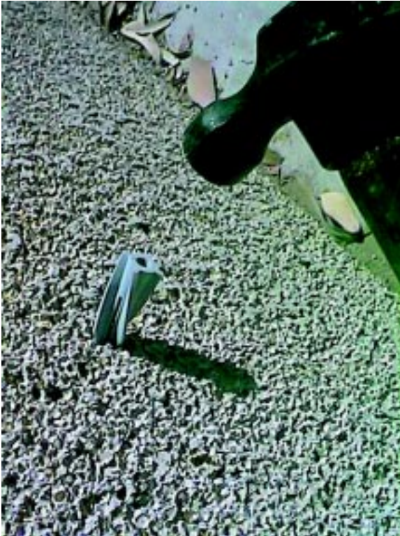
Figure 6.1 Setting anchor into RASTRA® element.
