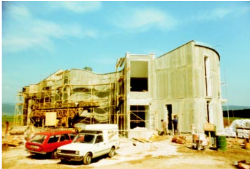
Figure 8.5 Office building ready for stucco finish.
