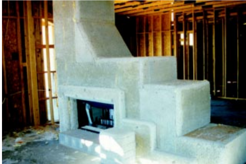
Figure 7.9 Zero-clearance fireplace coated with RASTRA® flat stock.
