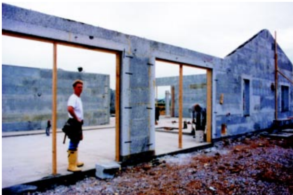
Figure 5.32 RASTRA® lintels with supports shortly after concrete pour.
