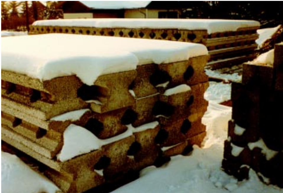
Figure B.6 Job site storage of RASTRA® elements.
