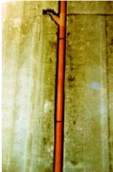
Figure A.7 Closeup of pipe installation.
