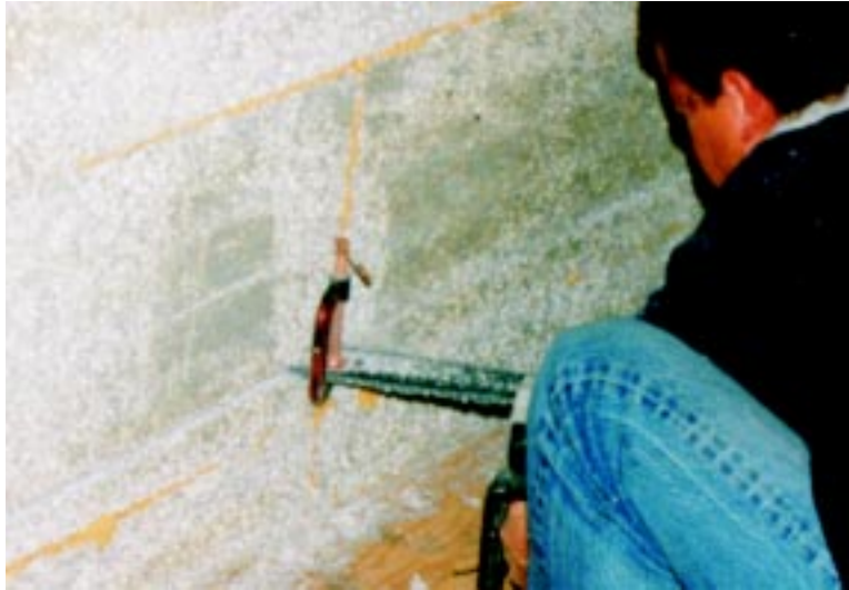
(a) Chain saw with C-clamp used as depth guide.
