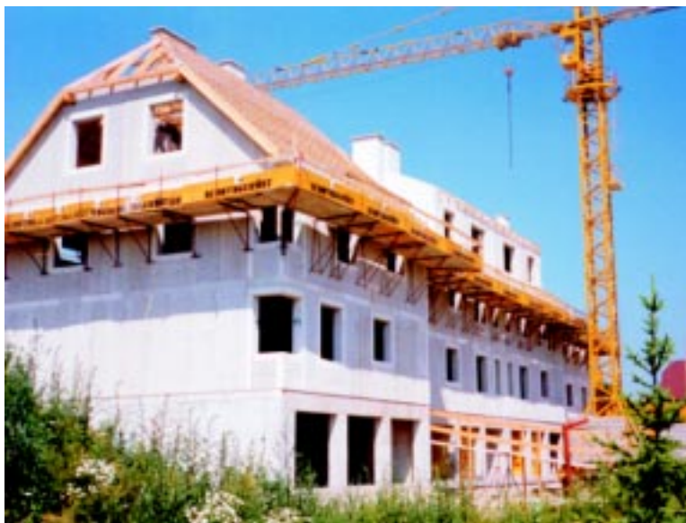
Figure 8.15 Prefabricated panels and window detail.
