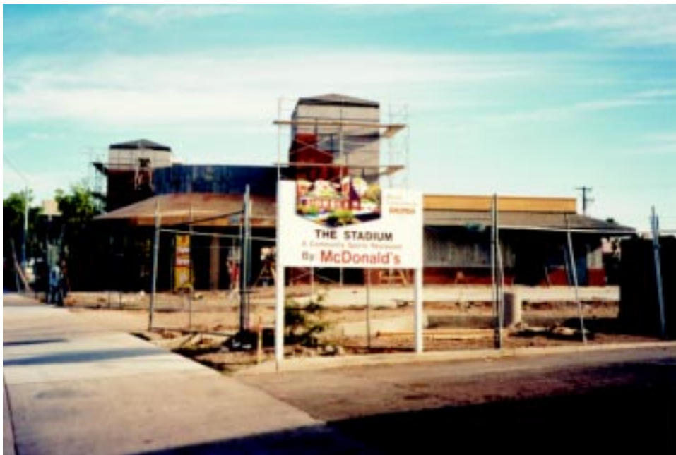
Figure 8.3 Tempe McDonald's under construction.
