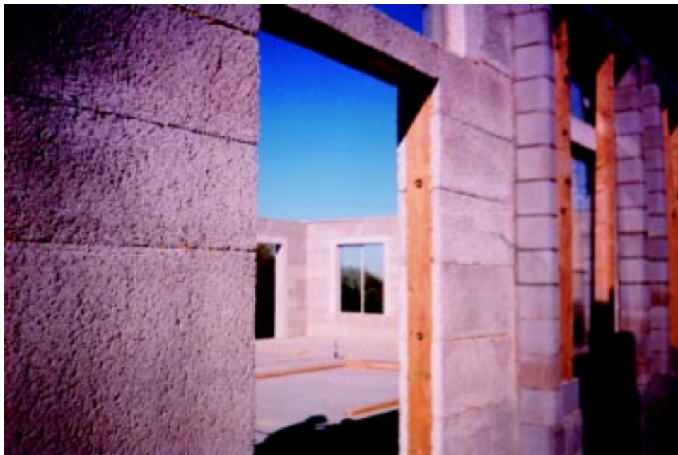
Figure 5.28 Recessed wood buck for swinging doors.
