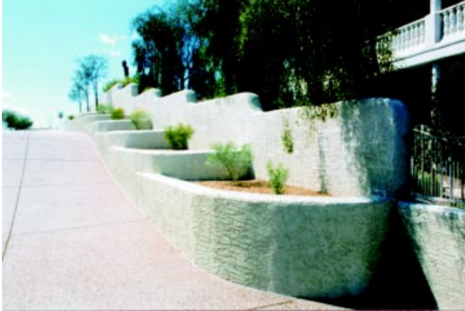
Figure 5.13 Curved planter and retaining wall.
