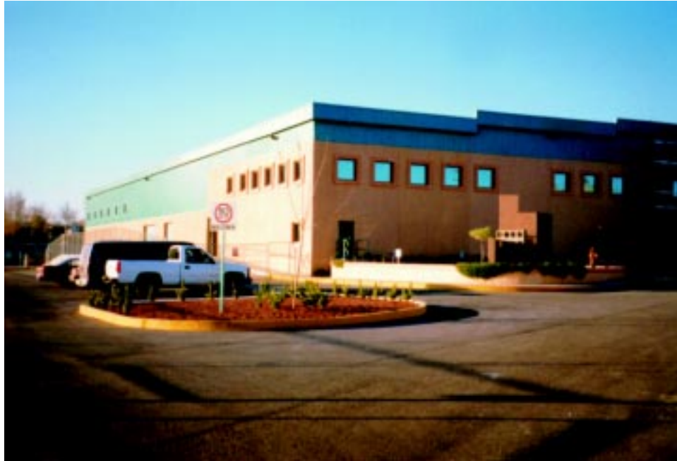
Figure 8.9 Painted exterior - 25ft high walls.
