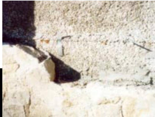
Figure 6.7 Brick veneer finish on RASTRA® home.
