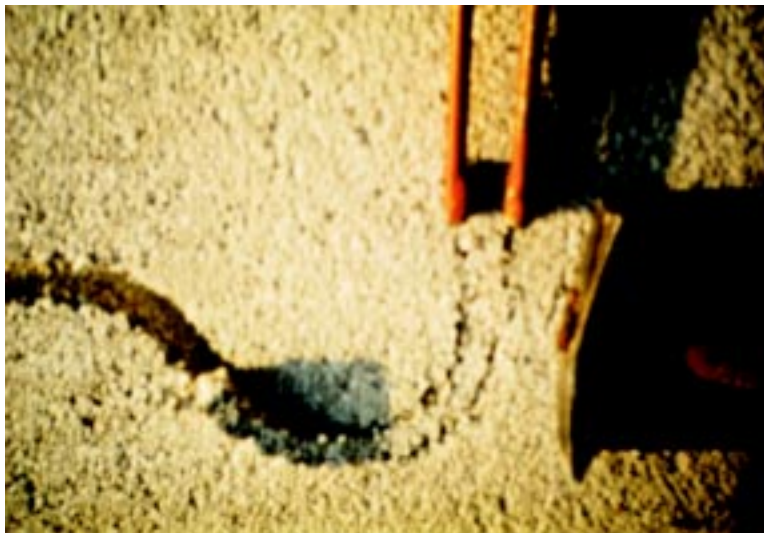
(b) Cutting groove with hand router.
