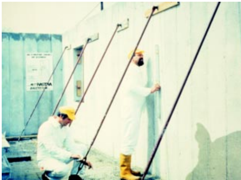
Figure 2.3 Turnbuckle adjusted to bring wall into plumb.
