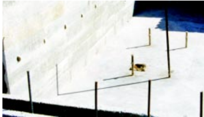
Figure 5.44 Grouting access holes.
