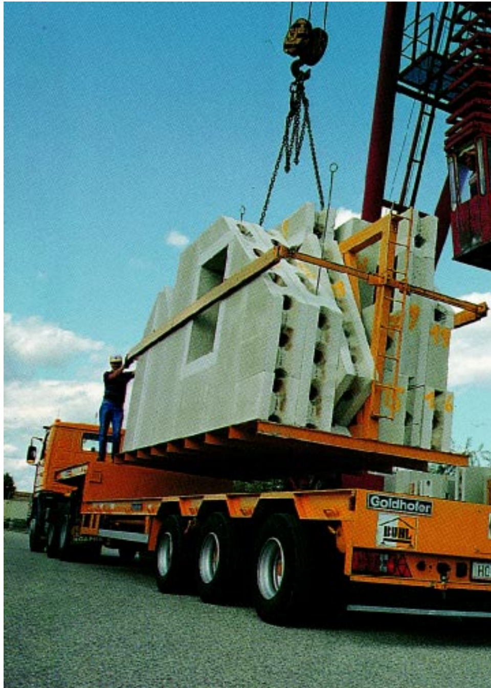
Figure 8.18 Prefabricated panel 14" thick.
