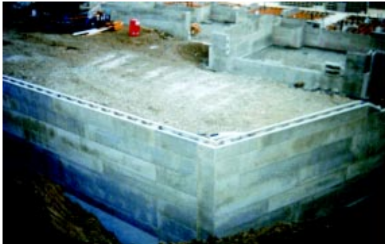
Figure 3.1 RASTRA® retaining wall prior to placement of vertical rebar, grouting and waterproofing.
