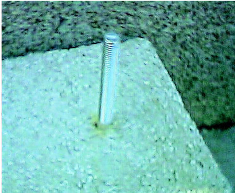
Figure 6.4 Threaded bolt for installing heavier items.
