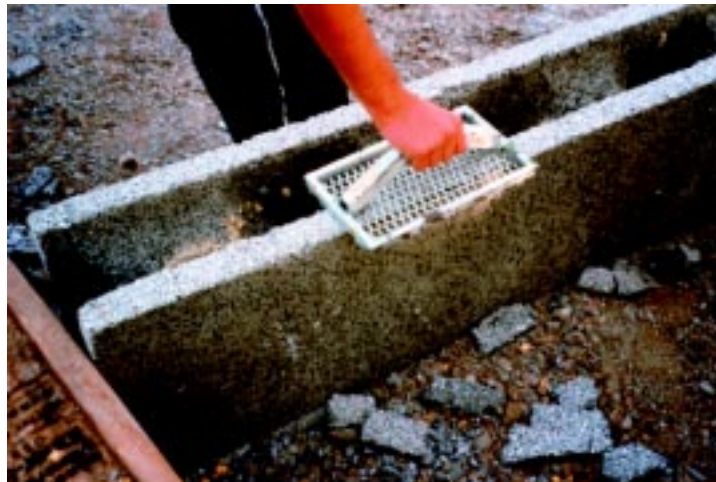
Figure 2.2 Shaping edge with hand rasp.
