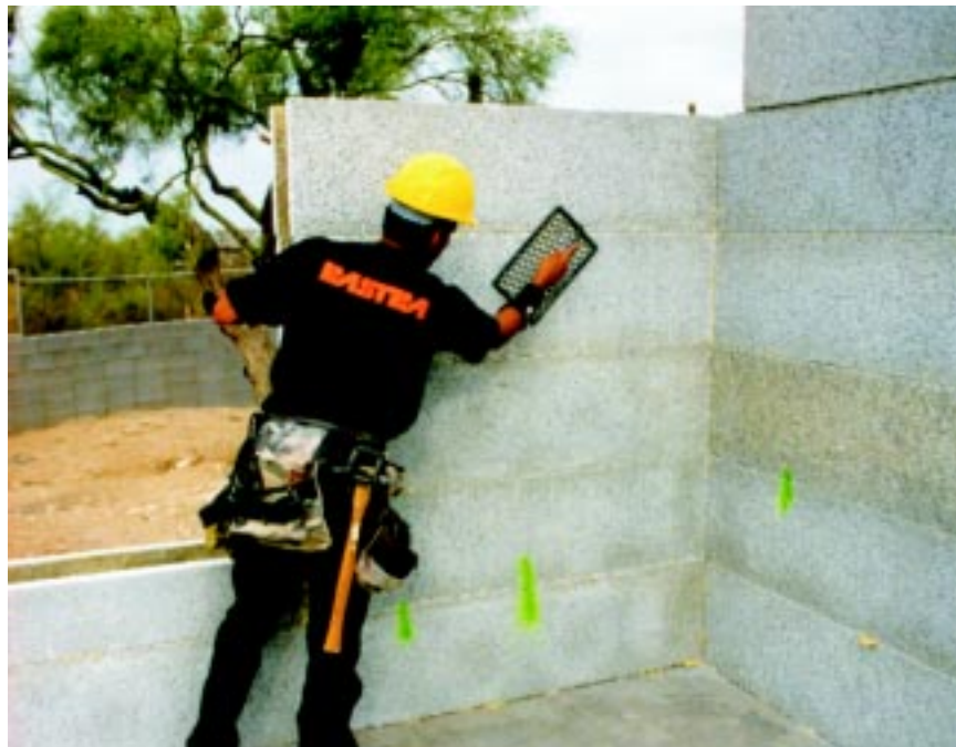
Figure 6.6 Rasping the interior surface.
