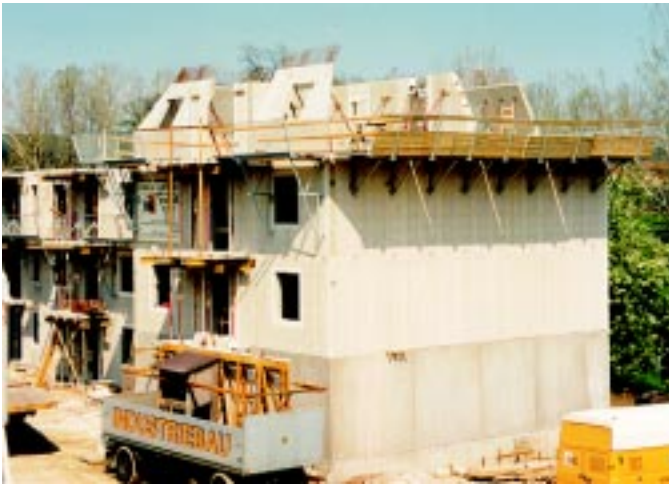
(a) Roof construction using RASTRA® prefabricated panels.
