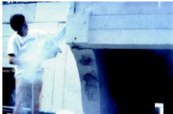
Figure 5.31 "Fine tuning" RASTRA® exterior.
