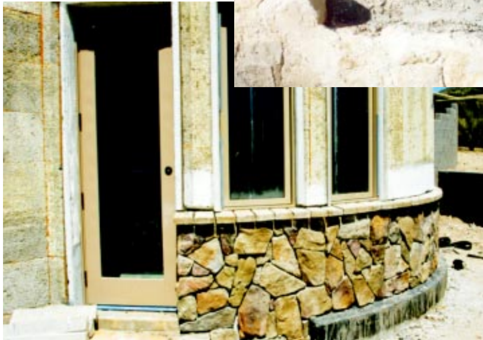
Figure 6.8 Veneer stone finish on curved RASTRA® wall. Insert shows wall ties.
