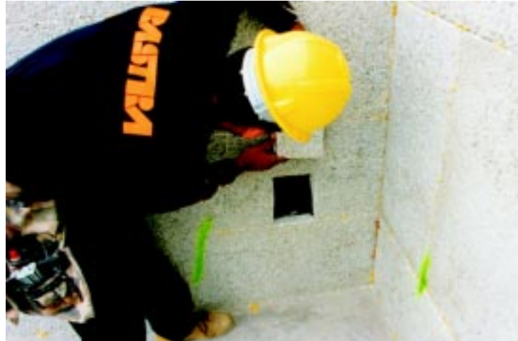
Figure A.8 Access hole for plastic pipe.
