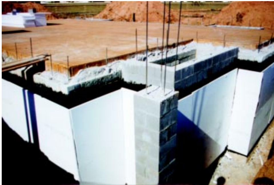
Figure 6.10 RASTRA® basement walls waterproofed and ready for backfilling.
