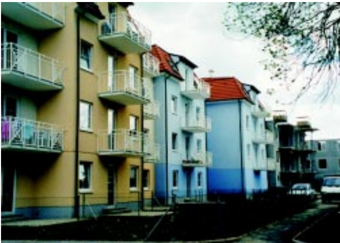
(c) Nearly completed complex.
