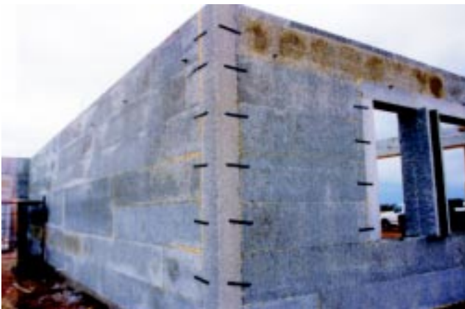
Figure 5.4 End element corner held in place with staples.
