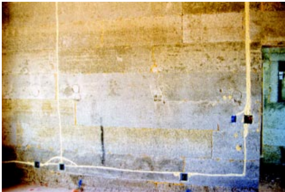
Figure A.2 Embedded wiring prior to plastering.
