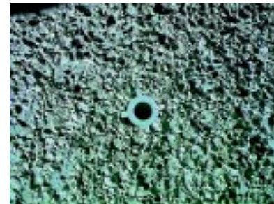
Figure 6.3 Closeup of embedded anchor.
