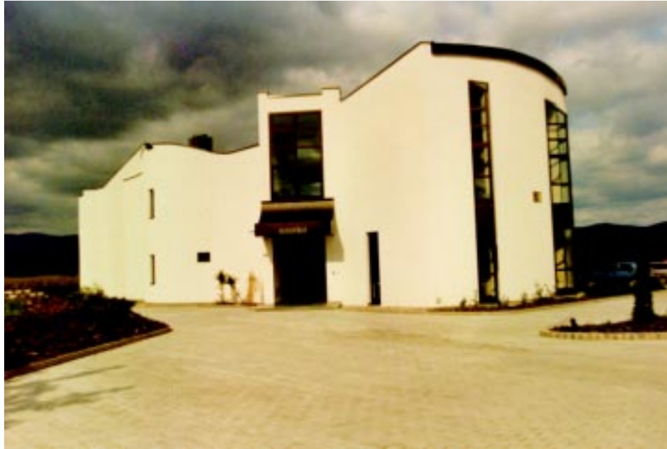
Figure 8.4 Completed 2-story office building.
