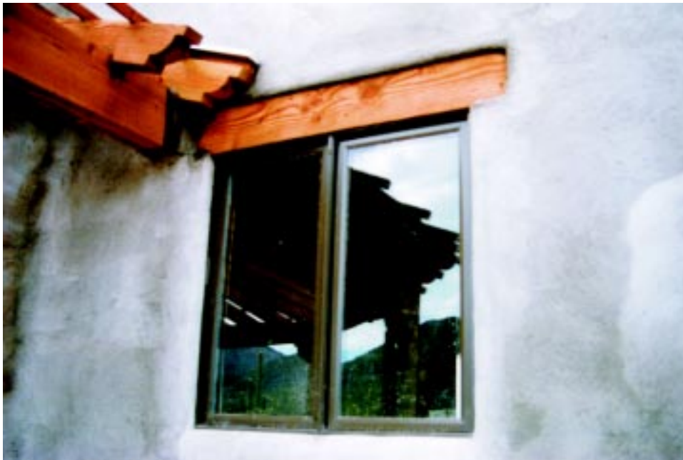
Figure 5.25 Wooden header - architectural detail.
