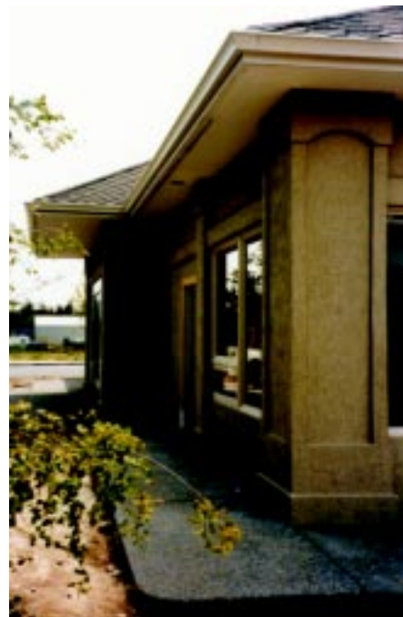
Figure 5.5 Millwork detail on house corner.
