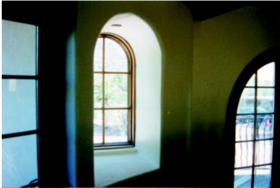
Figure 5.26 Custom window opening with deep sill and accent lighting.
