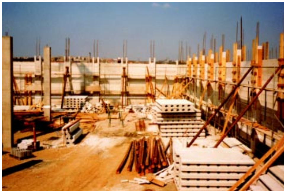
Figure 8.10 20ft upgoing Walls with Rastra Pillars
