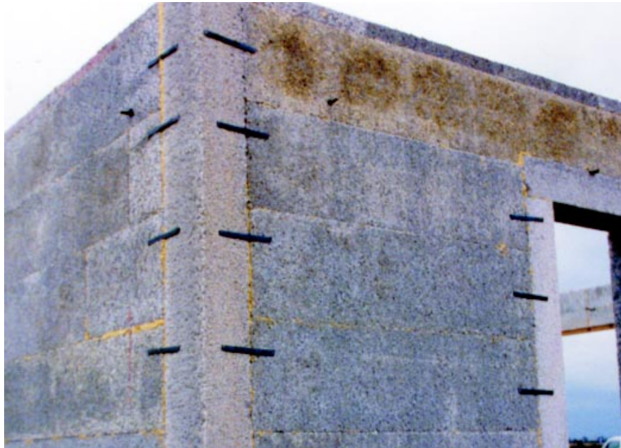
Figure 5.39 Standard elements laid horizontally and glued. End element installed vertically and stapled.
