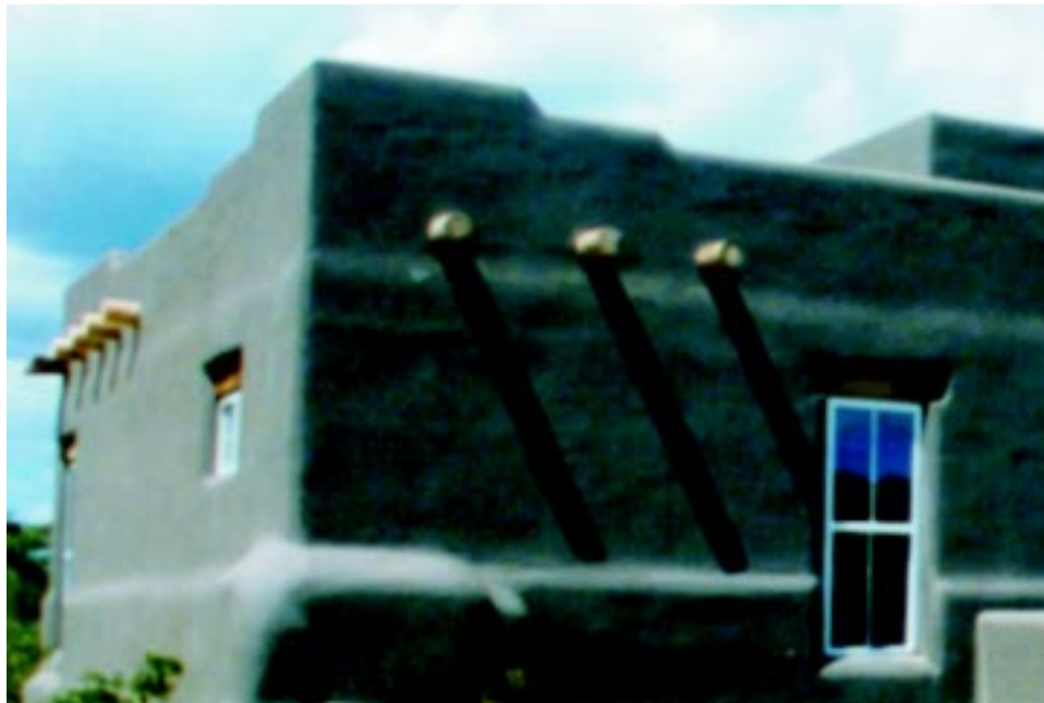
Figure 6.11 Southwest style home - flat roof & parapet.
