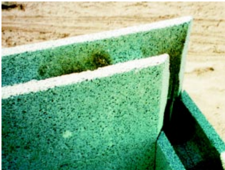
Figure 5.7 Corner made from standard elements cut to 45°.
