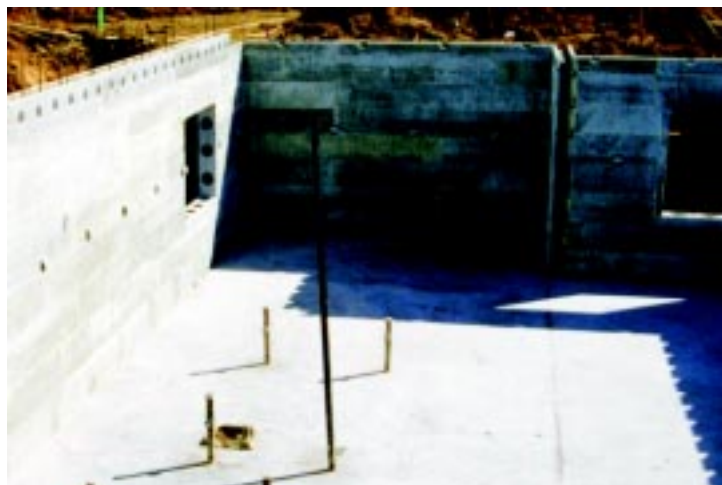
Figure A.9 Roughed-in plumbing.
