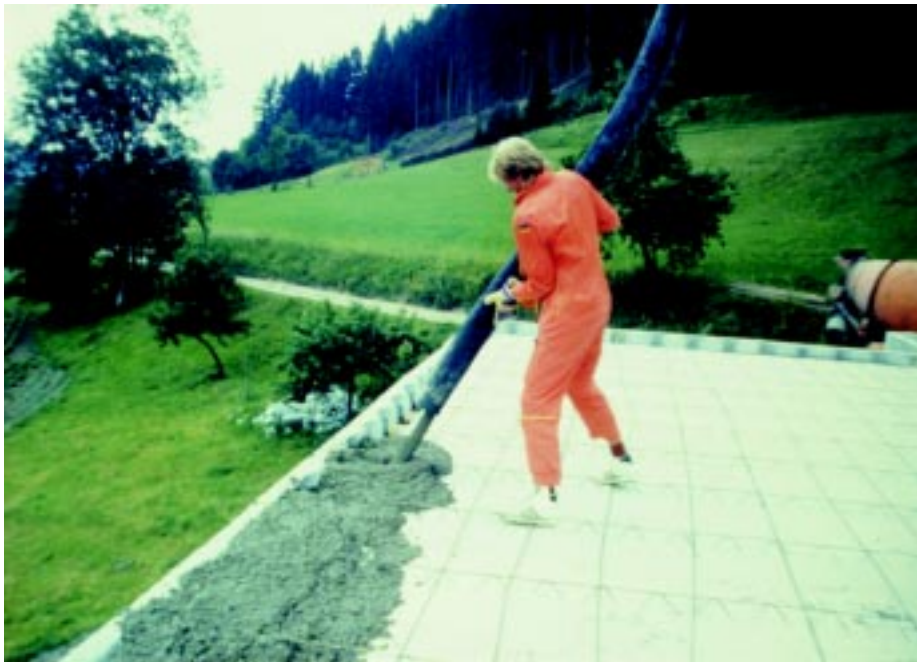
Figure 5.47 Grouting access holes.
