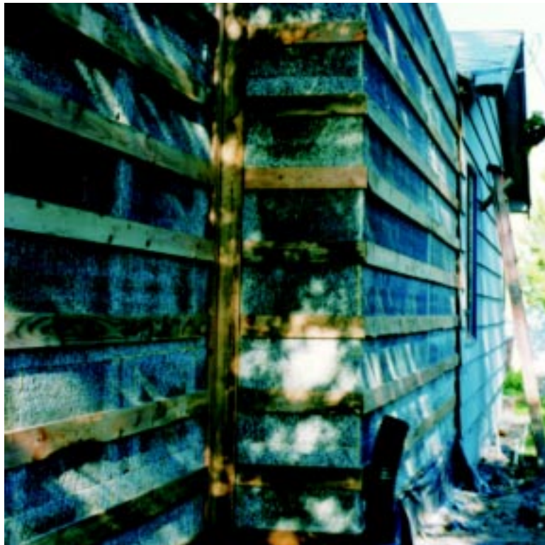
Figure 6.9 Nailers and siding on RASTRA® wall.
