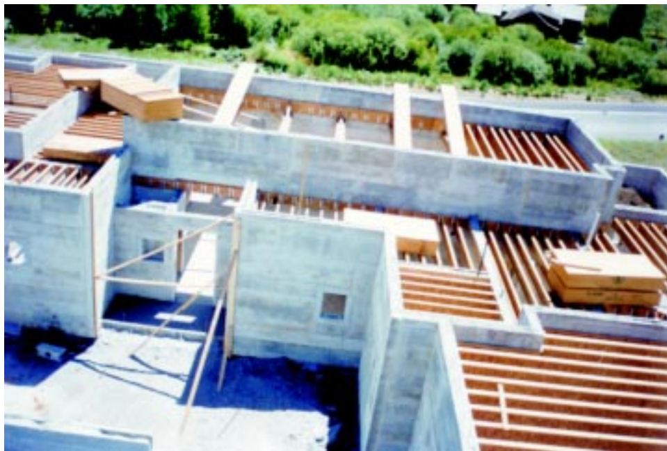
Figure 4.4 Installation of Truss-Joist system.
