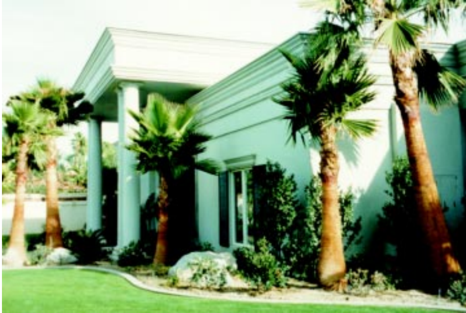
Figure 7.5 Home with RASTRA® walls, columns and molding.
