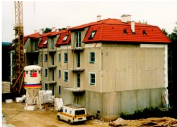
(b) Finished roof.
