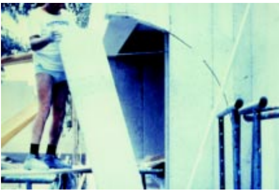
Figure 5.30 Trimming RASTRA® for curved support.
