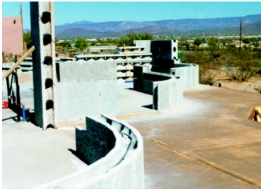
Figure 5.11 Curved walls under construction.
