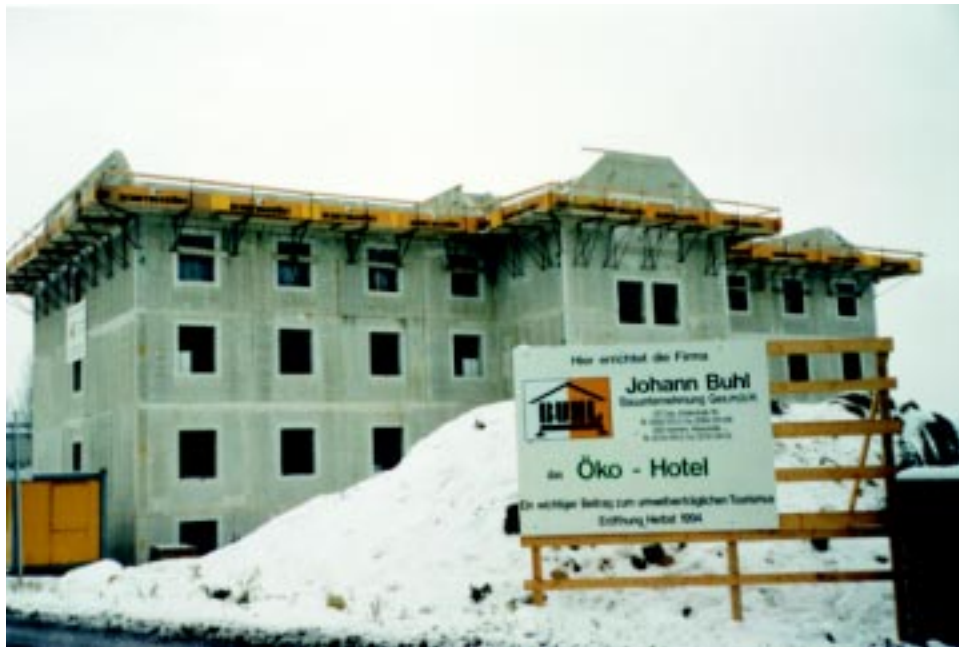
Figure 8.8 Front view of hotel - roof under construction.
