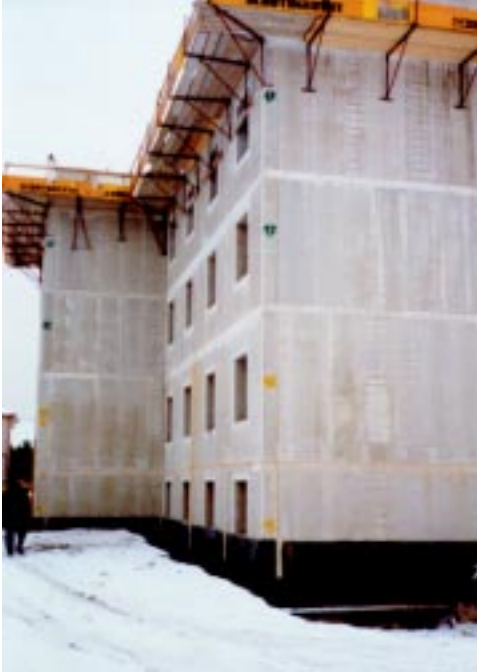
Figure 8.6 View of lower level waterproofing.
