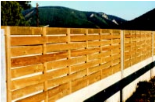
Figure 8.13 Sound wall with woven wood covering.
